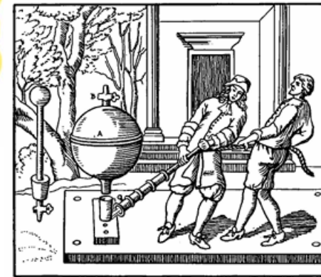
Fig. 2 The pumps of von Guericke in the 1640s. (Top) The first pump with a wooden barrel. (Bottom) The second pump with a copper sphere.
